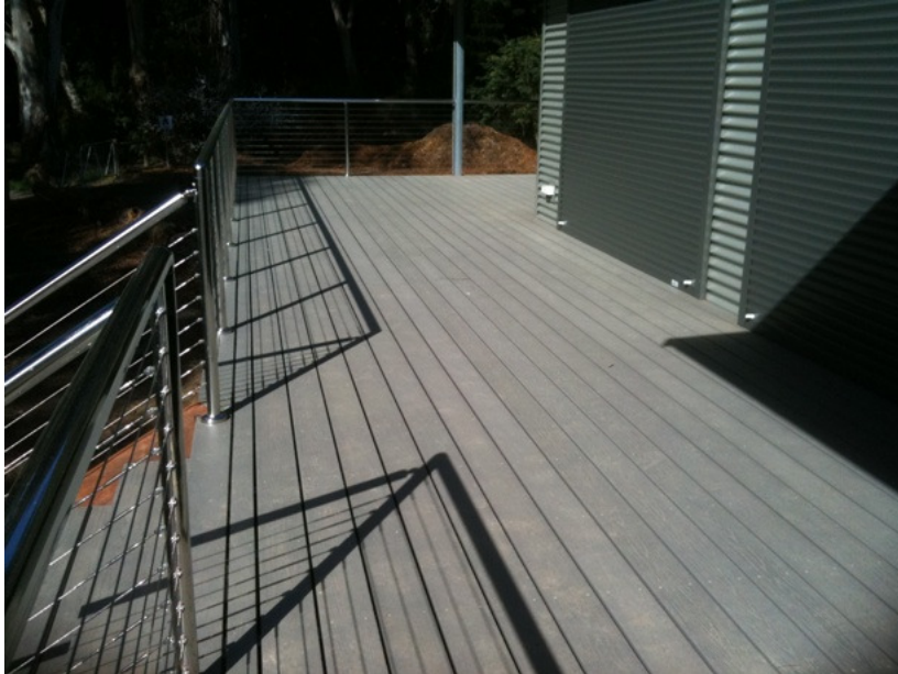
Murrindini Reserve Welcome Center deck in Australia
